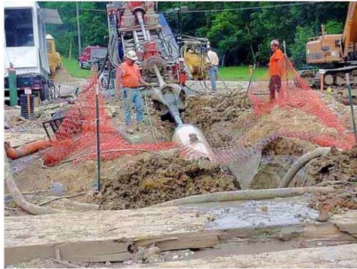
Figure 5. Typical mountain ridgeline construction
